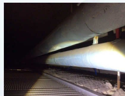
ITEM NO.: 12 PHOTO NO.: J161155-03-ISLHD-PKH-D-PHOTO010 RESULT: SMF - PRESUMED POSITIVE BUILDING/LEVEL: DENTAL & CHILDCARE - LEVEL 01 ROOM/LOCATION: CORRIDOR - CEILING SPACE FEATURE/MATERIAL: INSULATION BATTS - INSULATION MATERIAL SAMPLE NO.: -
