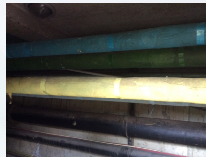
ITEM NO.: 8 PHOTO NO.: J161155-03-ISLHD-PKH-D-PHOTO016 RESULT: SMF - PRESUMED POSITIVE BUILDING/LEVEL: DENTAL & CHILDCARE - LEVEL 00 ROOM/LOCATION: SUBFLOOR - RUNNING NORTH SOUTH FEATURE/MATERIAL: PIPEWORK INSULATION - INSULATION MATERIAL SAMPLE NO.: -
