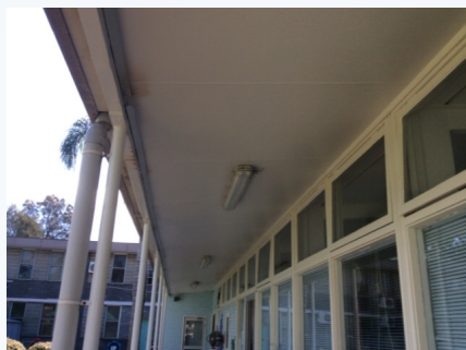
ITEM NO.: 1 PHOTO NO.: J161155-03-ISLHD-PKH-D-PHOTO004 RESULT: ASBESTOS - PREVIOUSLY SAMPLED NEGATIVE BUILDING/LEVEL: DENTAL & CHILDCARE - LEVEL 00 ROOM/LOCATION: PLAYGROUND PKBD0039 - SOUTHWEST FEATURE/MATERIAL: AWNING - FIBRE CEMENT SHEETING SAMPLE NO.: PREVIOUSLY SAMPLED GREENCAP J149255-03-PKDH - D-002
