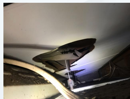
ITEM NO.: 6 PHOTO NO.: J161155-03-ISLHD-PKH-D-PHOTO019 RESULT: ASBESTOS - PRESUMED POSITIVE BUILDING/LEVEL: DENTAL & CHILDCARE - LEVEL 00 ROOM/LOCATION: PLAYRM PKBD0011 - WEST CEILING SPACE FEATURE/MATERIAL: CEILING ABOVE SUSPENDED CEILING - FIBRE CEMENT SHEETING SAMPLE NO.: PREVIOUSLY SAMPLED GREENCAP SIMILAR TO J149255-03-PKDH - D-001
