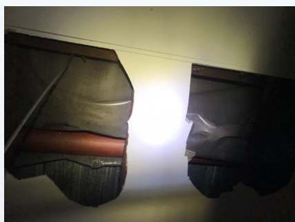
ITEM NO.: 5 PHOTO NO.: J161155-03-ISLHD-PKH-D-PHOTO020 RESULT: ASBESTOS - PREVIOUSLY SAMPLED POSITIVE BUILDING/LEVEL: DENTAL & CHILDCARE - LEVEL 00 ROOM/LOCATION: OFFICE PKDB0012 - CEILING SPACE FEATURE/MATERIAL: CEILING ABOVE SUSPENDED CEILING - FIBRE CEMENT SHEETING SAMPLE NO.: PREVIOUSLY SAMPLED GREENCAP J149255-03-PKDH - D-001
