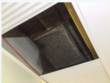
ITEM NO.: 11 PHOTO NO.: J161155-03-ISLHD-PKH-D-PHOTO011 RESULT: SMF - PRESUMED POSITIVE BUILDING/LEVEL: DENTAL & CHILDCARE - LEVEL 01 ROOM/LOCATION: CEILING SPACE - THROUGHOUT FEATURE/MATERIAL: INSULATION BATTS - INSULATION MATERIAL SAMPLE NO.: -
