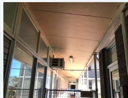
ITEM NO.: 2 PHOTO NO.: J161155-03-ISLHD-PKH-D-PHOTO018 RESULT: ASBESTOS - PRESUMED NEGATIVE BUILDING/LEVEL: DENTAL & CHILDCARE - LEVEL 00 ROOM/LOCATION: VERANDAH EAST - THROUGHOUT FEATURE/MATERIAL: CEILING - FIBRE CEMENT SHEETING SAMPLE NO.: PREVIOUSLY SAMPLED GREENCAP SIMILAR TO J149255-03-PKDH - D-002
