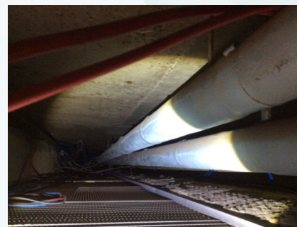
ITEM NO.: 4 PHOTO NO.: J161155-03-ISLHD-PKH-D-PHOTO007 RESULT: SMF - PRESUMED POSITIVE BUILDING/LEVEL: DENTAL & CHILDCARE - LEVEL 00 ROOM/LOCATION: CORRIDOR INT PKBD0005 - CEILING SPACE FEATURE/MATERIAL: PIPEWORK INSULATION - INSULATION MATERIAL SAMPLE NO.: -
