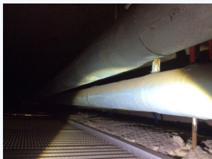
ITEM NO.: 3 PHOTO NO.: J161155-03-ISLHD-PKH-D-PHOTO008 RESULT: SMF - PRESUMED POSITIVE BUILDING/LEVEL: DENTAL & CHILDCARE - LEVEL 00 ROOM/LOCATION: CORRIDOR INT PKBD0005 - CEILING SPACE FEATURE/MATERIAL: INSULATION BATTS - INSULATION MATERIAL SAMPLE NO.: -
